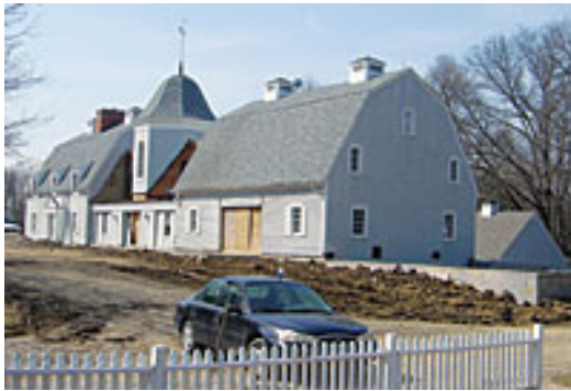
These three barns were put together to form a 12,000-square-foot home. This is the pre-construction phase, prior to the roofline's change and major construction.
